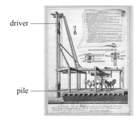
(a) (i) The driver on the pile driver above had a mass of 810 kg and could be dropped a maximum distance of 6.0 m onto the pile.
